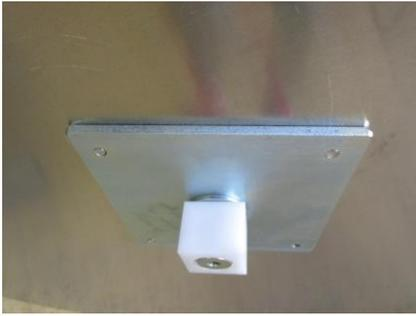
Stick 1 washer  $\varnothing$  outside 44 mm, DIN 126 and then 1 polyamide liner 40 x 40 mm on the plugs.
