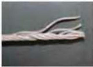
FRAYED Cable strands visible & unraveling
