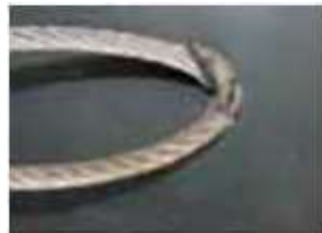
CRIMPED Gaps in the strands where the cable was crimped
