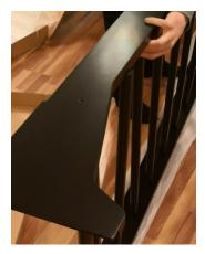
Fit the second rail on the top of the oval bars. Start at one end and progressively insert oval bars until all are seated. Use wooden block and rubber mallet if necessary to fully seat oval bars. Be careful not to damage or scratch the surface. Screw three oval bars to the
