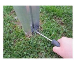
b) Set mounted goal with fixed ground sockets in the foundations (80x80x100cm). To enable a drain off of possible water we recommend to stick a tube each below the boreholes of the ground sockets. After careful adjustment of the goal to the side and specified height by crossed bars pour concrete into the foundation ditches. Do not apply an accelerating mixture or antifreeze as these adhesives may cause damages of ground sockets.
